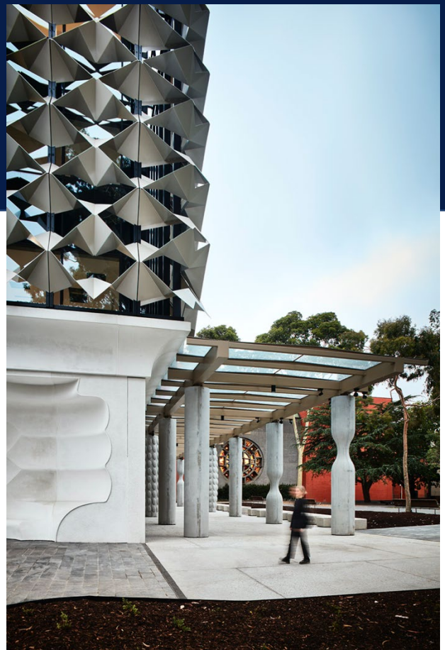
Monash University Chancellery Building
